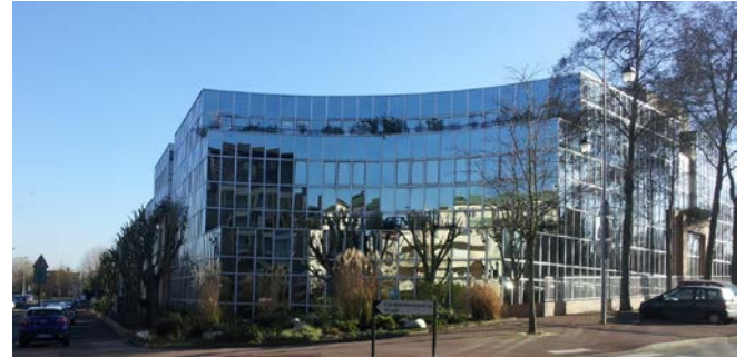
IALA Headquarters, Saint-Germain-en-Laye, France
