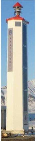
While typical results for NCA05 natural frequency analysis averaged around **6.15 Hz** at positive temperatures, it increased to **6.69 Hz** in above case and even **7.4 Hz** below **-10°C**
