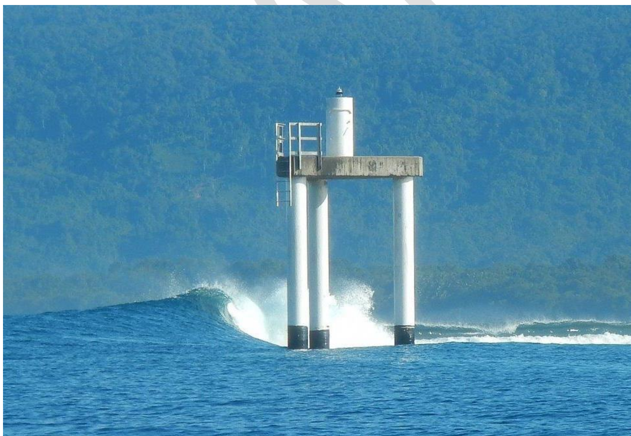
Figure 2 Example of multi-steel piled, concrete light platform with GRP light tower, access ladder and tape wrapped piles within the splash zone
