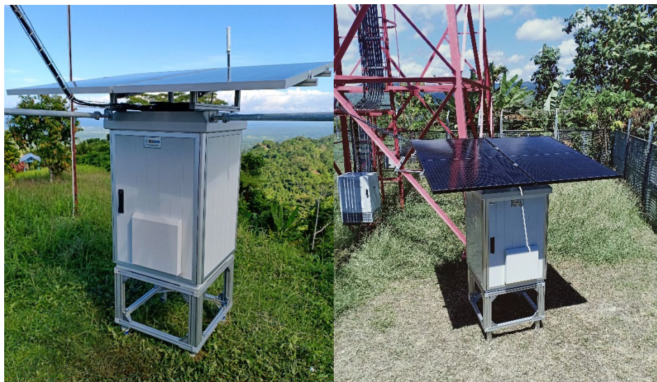
Figure 84: AIS Coastal Station Enclosure
