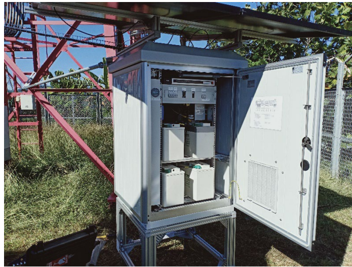
Figure 85: AIS Coastal Station Enclosures (Battery Array and AIS Base Station)
