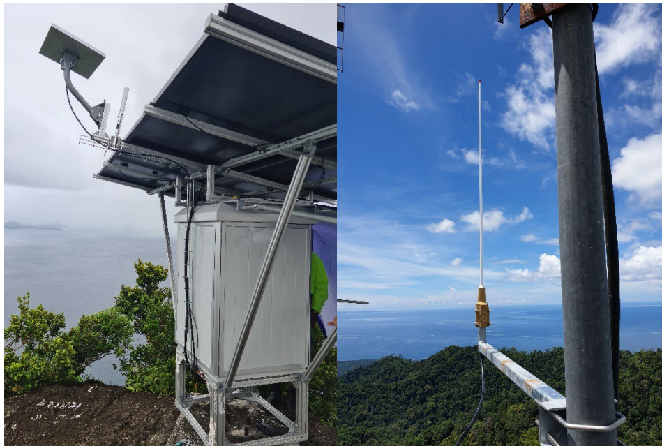
Figure 86: AIS Coastal Station Enclosure; BGAN Terminal and VHF Antenna
