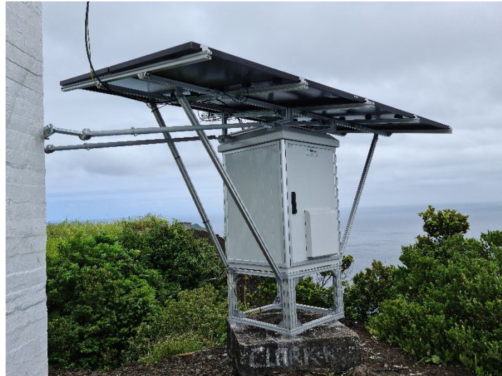
Figure 83: AIS Coastal Station Enclosure
