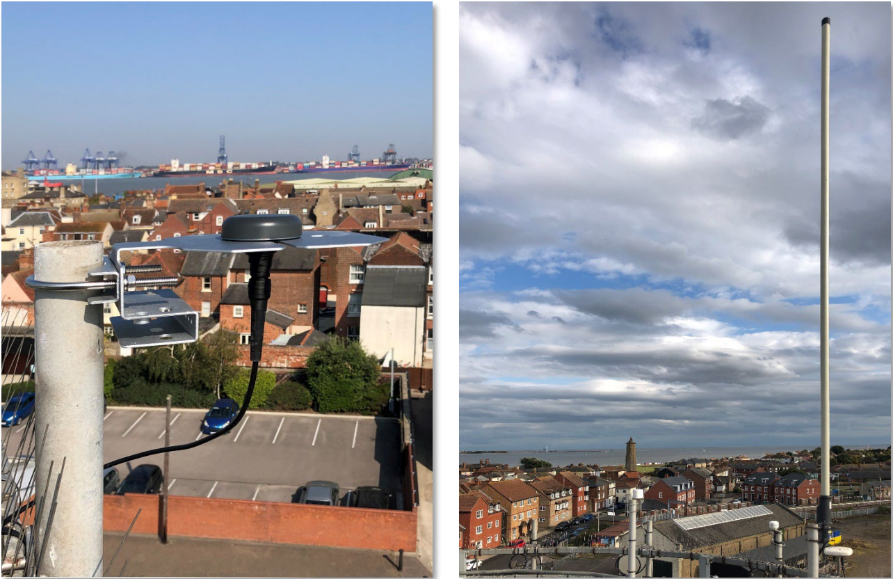
Figure 99: GNSS (left) and VHF Antenna installation on the TH Buoy Yard Building 'rotunda'.
