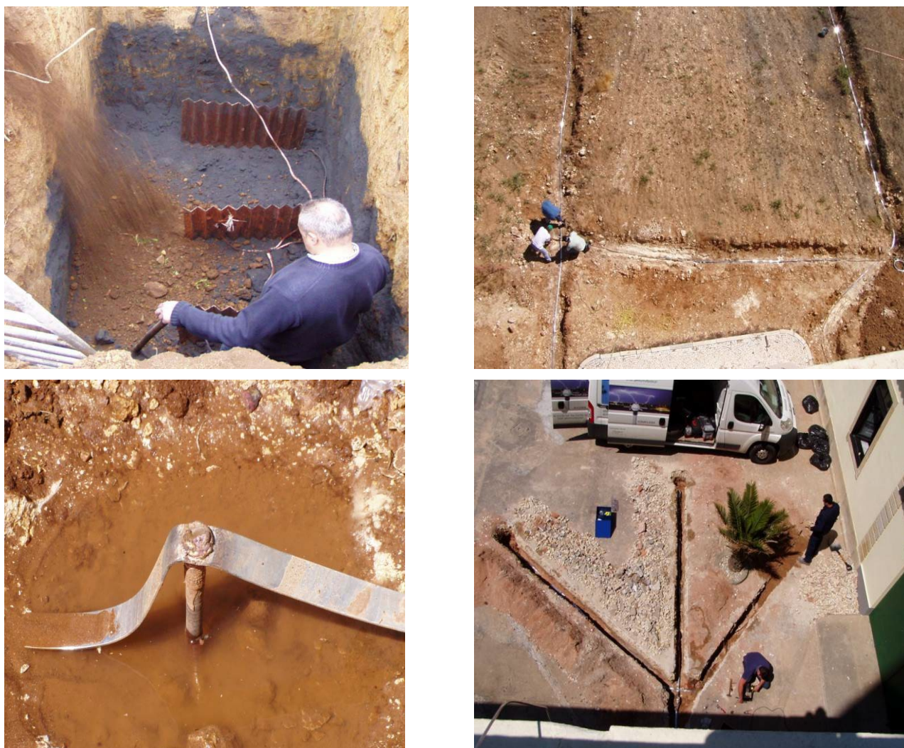
Figure 19 Different types of earth electrodes
