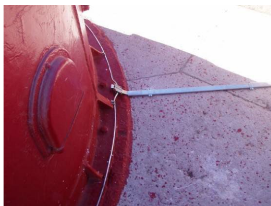
Figure 14 An example of murette bonding
