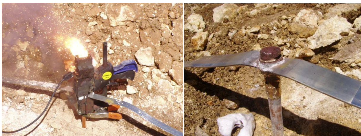
Figure 20 Aluminothermic Welding
