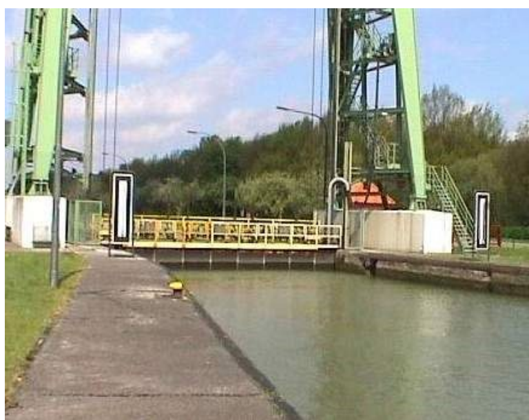
Figure 13 Entrance lock navigation aids (Germany) can be seen to the left and right of the lock gate
