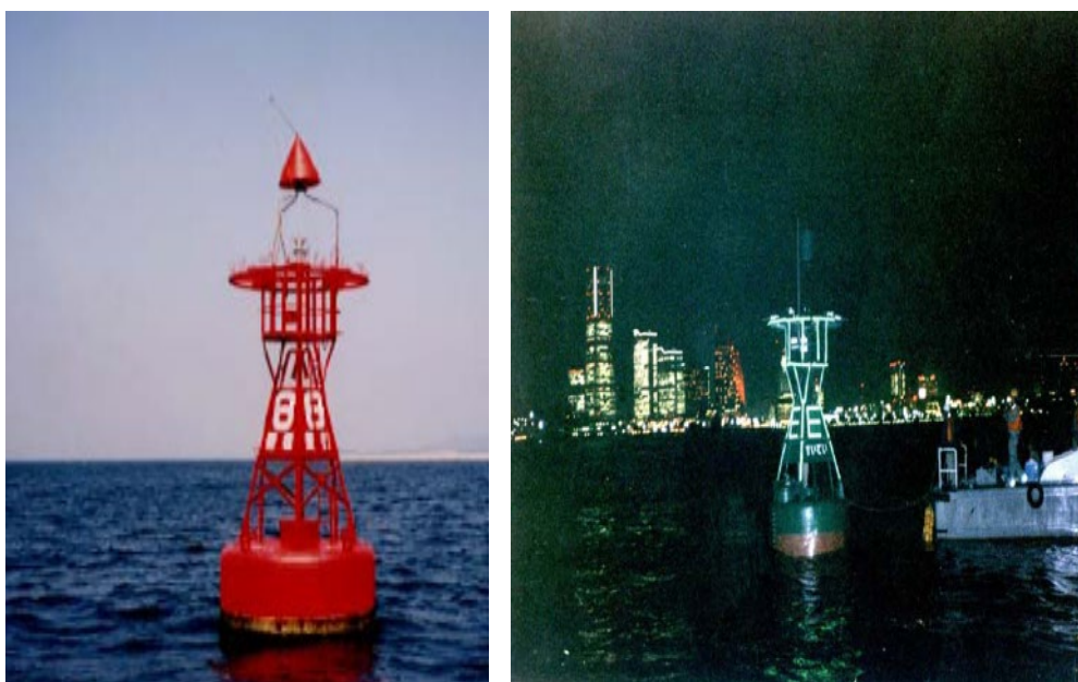
Figure 9 Contour lighting on a floating aid, Japan
