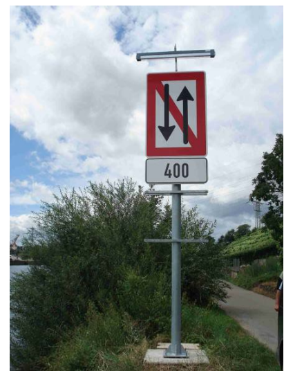
Figure 15 Typical sign with luminaire at the top (Germany)
