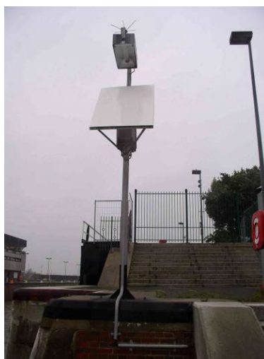
Figure 7 Plate size: 1050 x 760 mm: low pressure sodium lamp 90W
