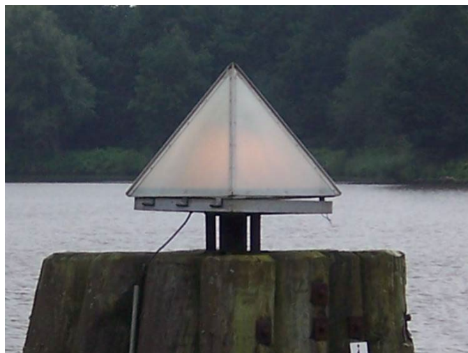
Figure 8 An acrylic pyramid illuminated from the inside to mark a dolphin
