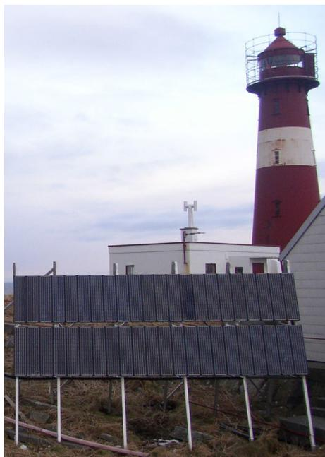
Figure 2 *Grasøyane lighthouse solar array*
