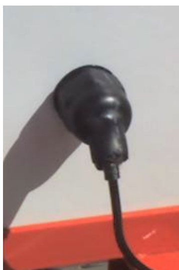
Figure 19 Sealed cable gland with heat shrink
