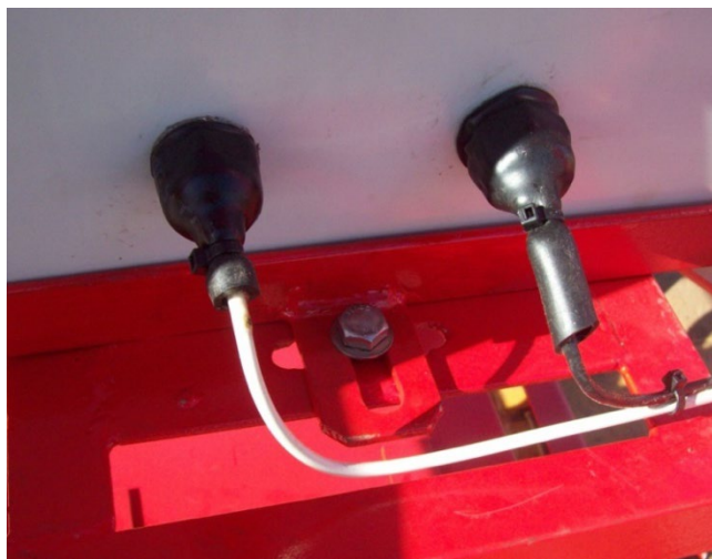
Figure 18 Sealing of antenna and power supply inputs.
